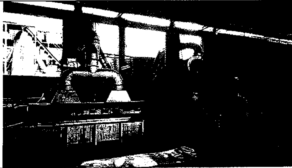
Installation of Fume absorber for control of Acid Fumes in Rolling & Pickling Units
